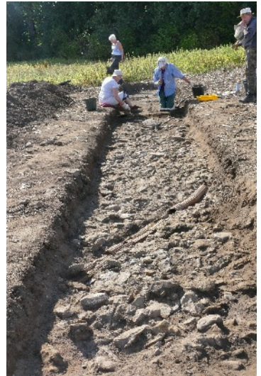
Watling Street Foundations on the road
